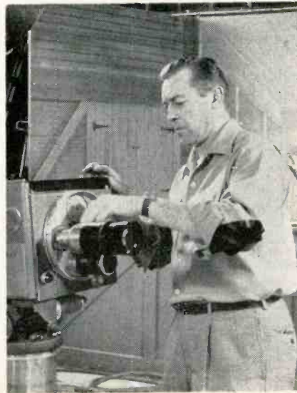
Fig. 7: Removing the camera lens turret
