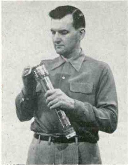
Fig. 4: Use lens tissue to clean tube face
