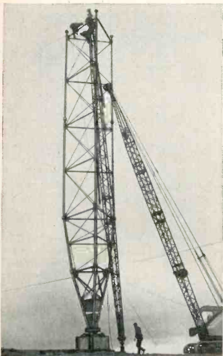
Construction close-up on new 1282-foot Truscon Triangular Guyed Tower for WTV in Cadillac, Mich.
